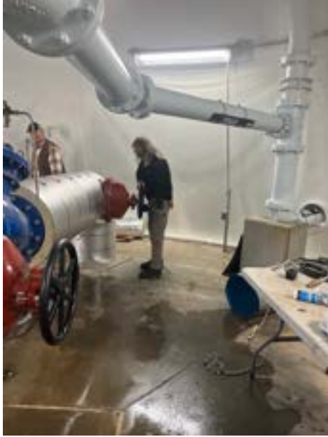
Figure 7 - Harrington Water Upgrades
