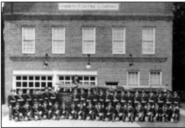
Figure 4 - Old Harrington Fire Department
