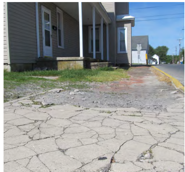
Downtown sidewalk in a predominantly residential area in need of repair.
