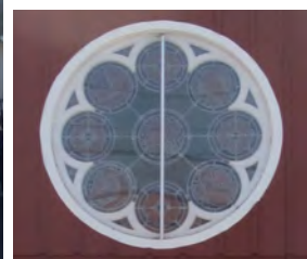
St. Stephen's Church, as it now looks, is used as part of the Harrington Historical Society complex. As of April 2016, it is the only property in the City of Harrington that is listed on the National Register of Historic Places.
