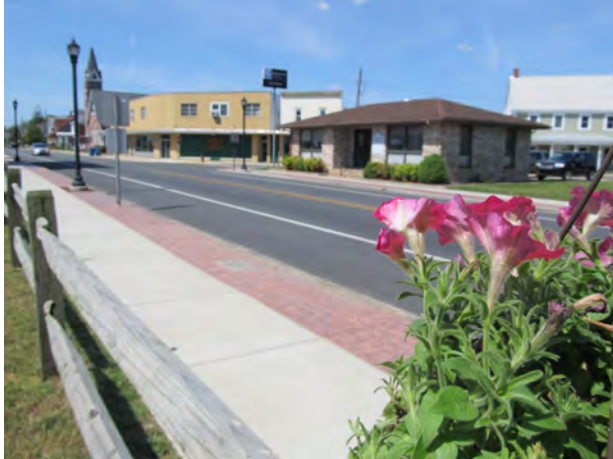
Sidewalk in a predominantly commercial area that has been improved as part of the Downtown Streetscape Improvement project.
