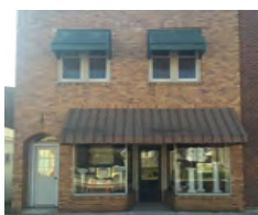
Clark Street two-story vacant building next to Bowers Group, formerly an antique retail store.
