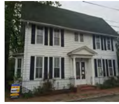
Single-family two story residential structure located at 19 Dorman Street.
