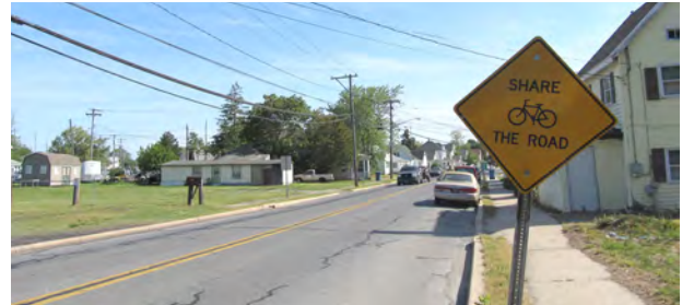
Delaware Avenue, near the Downtown boundary. A “Share the Road” sign has good intentions; however, a designated bike lane or shared lane markings would be more beneficial. Delaware Avenue is a State-maintained and regulated roadway.
