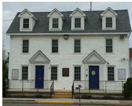
Harrington's City Hall, located at 106 Dorman Street, has recently undergone renovations, both to its interior and its exterior.
