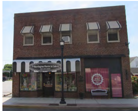
The Harrington Florist & Cakery, before (left) and after (right), with a new facade. Changes include new signage, paint, and awnings.
